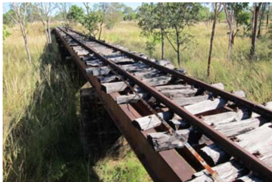
Trestle Bridge and NAR Corridor, Katherine
