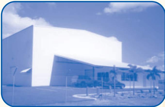
Pickfords Records Management building, Darwin
