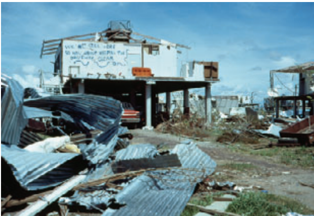
LEO JOHN ADAMS, NTRS 3128, Reference copy of digitised images of slides relating to Cyclone Tracy, 1974, Item 30, Sign on Casuarina house [view of cyclone damaged house, sign reads "we're still here so how about keeping the driveway clear"], 26/12/1974
