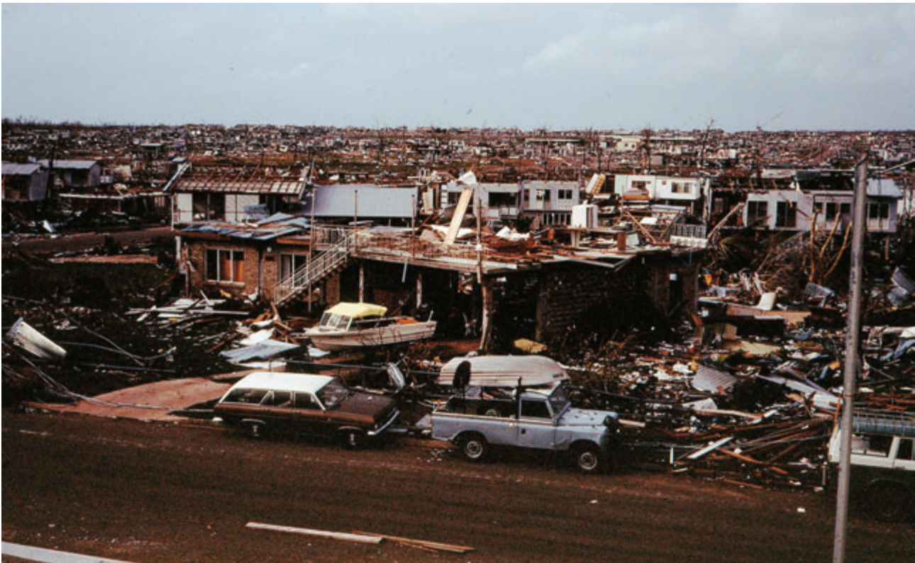
LEO JOHN ADAMS, NTRS 3128, Reference copy of digitised images of slides relating to Cyclone Tracy, 1974, Item 4, Alawa [view of cyclone damaged houses], 25/12/1974
